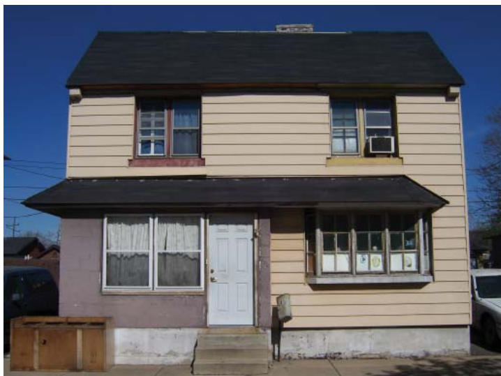
Image 6: Some of the stucco facades have been reclad with inappropriate finishes. Above, this home was covered with aluminum siding. The porch has been enclosed and the door style is inappropriate.
