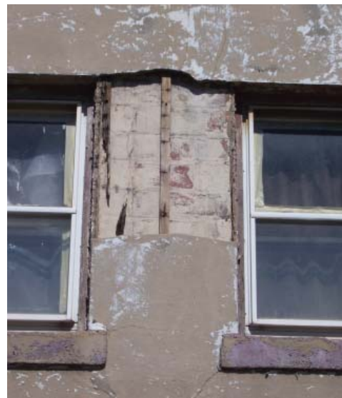
Image 4: The above image shows the extreme deterioration of some of the stucco facades.
