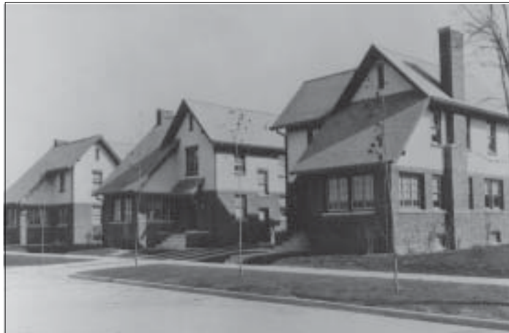
While only three Supervisor's Homes were completed, both sides of Broad Street were to have been lined with these classic Howard Shaw designs. Each home had its own garage and all were separated from the worker homes by a brick garden wall. C.1920
