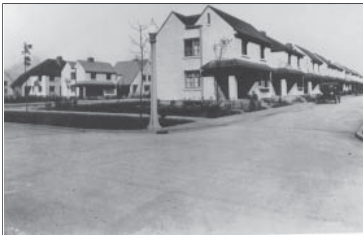
Park Street at Pine Avenue. Note the original cast concrete light post at the corner. When Marktown was first built, the only fences were the two concrete fences on the 500 block of Lilac Street. Note the open porches which actually increased the level of security for each home. Circa 1920.
