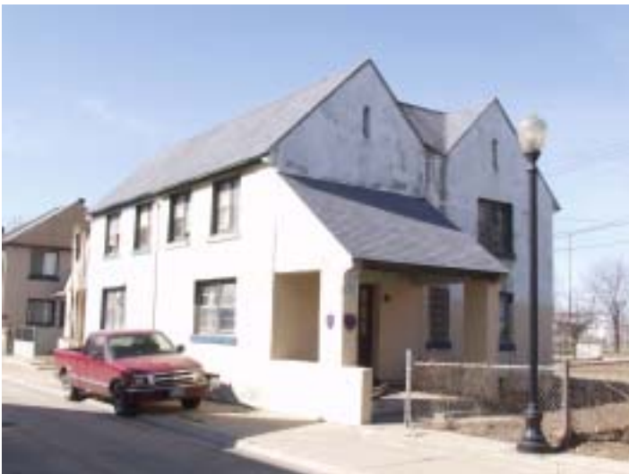
410-412 Prospect Street - A Work In Progress
