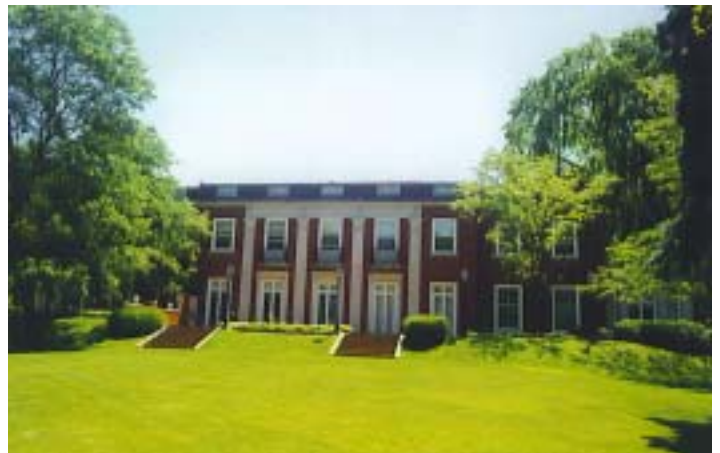
Erskine Estate - South Bend, Indiana
