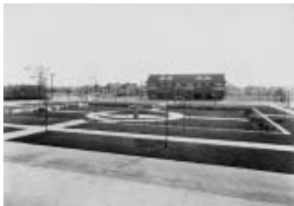
The Yellowstone Trail passed on both sides of the Marktown Market Square fountain and park. The park was removed for public safety reasons in 1936. One small section of the original street still exists just across from Mr. Shaw's 1917 Market Square building.
