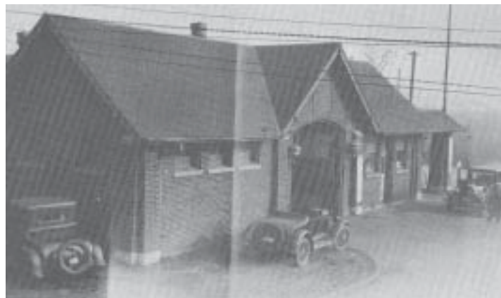
The original Marktown Garage which services company and Marktown resident vehicles. Now Michels Bar & Grill
