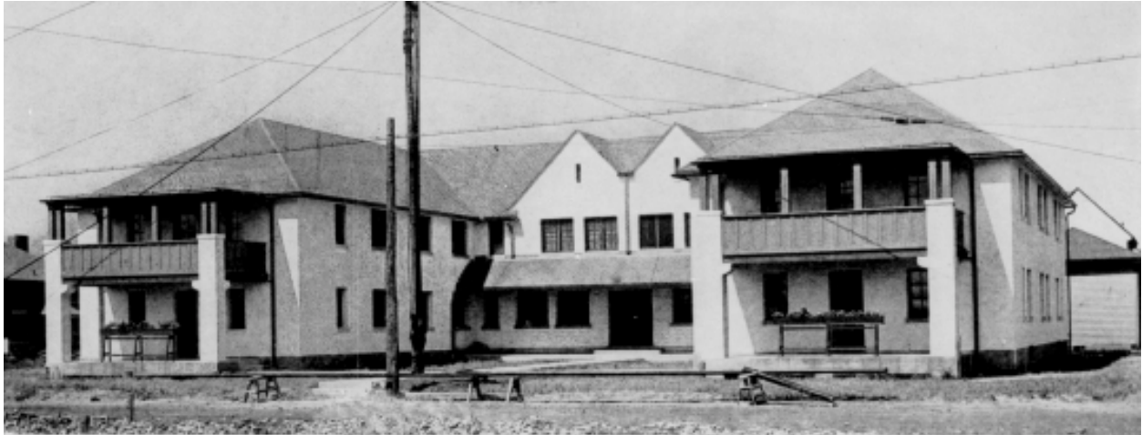
View of Boarding House
