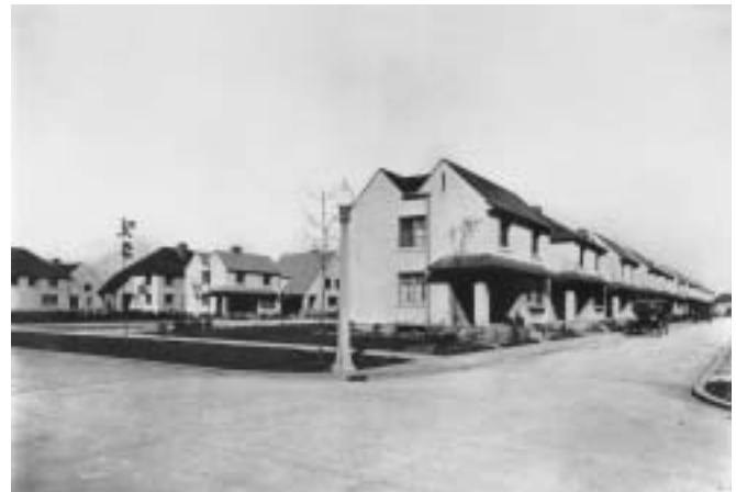
And with that work force came the need for modern, quality housing for their workers and families!
