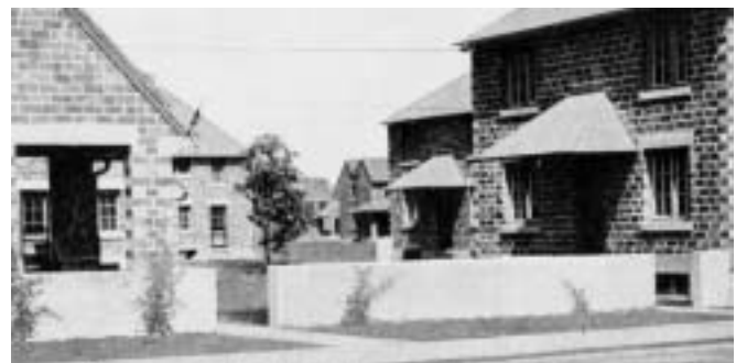
Marktown during construction in 1918. The photo was not a part of the original article.
