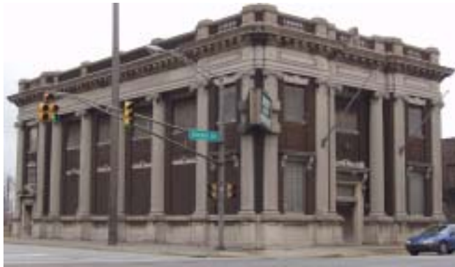
Above: Will we save the Riley Bank by finding a new use for this grand old structure? We definitely hope so!
