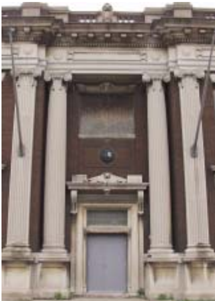
Above: The classic entrance way to the bank is flanked by Ionic columns and pilasters executed in Indiana Bedford limestone.
