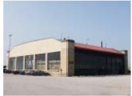
Ford Hangar in Lansing
