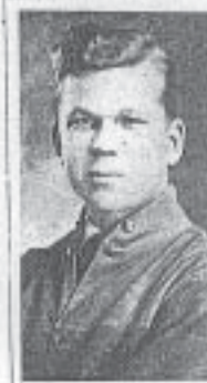
Oscar Frazier, a crane-man in the Hot Mills.
